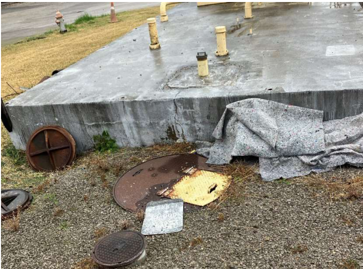
Photo 1: 10,000-Gallon UST (most under concrete slab)
