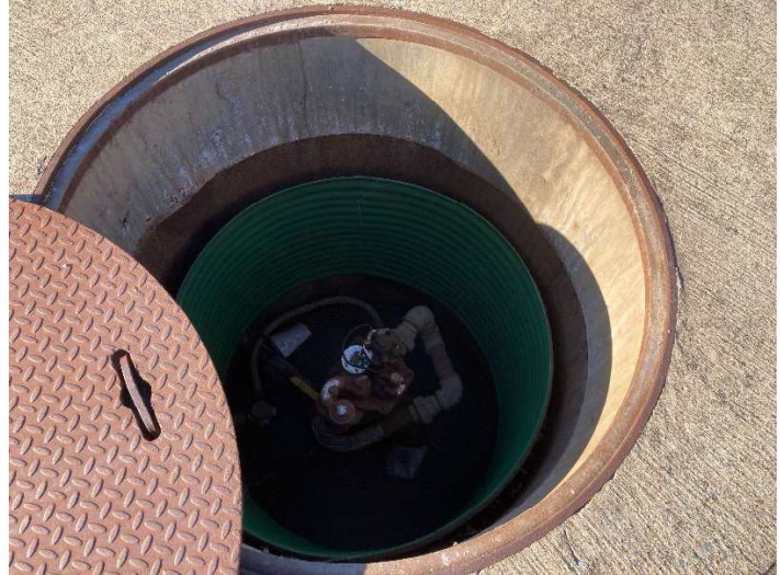
Photo 4: 20,000-Gallon UST Pump Manhole
