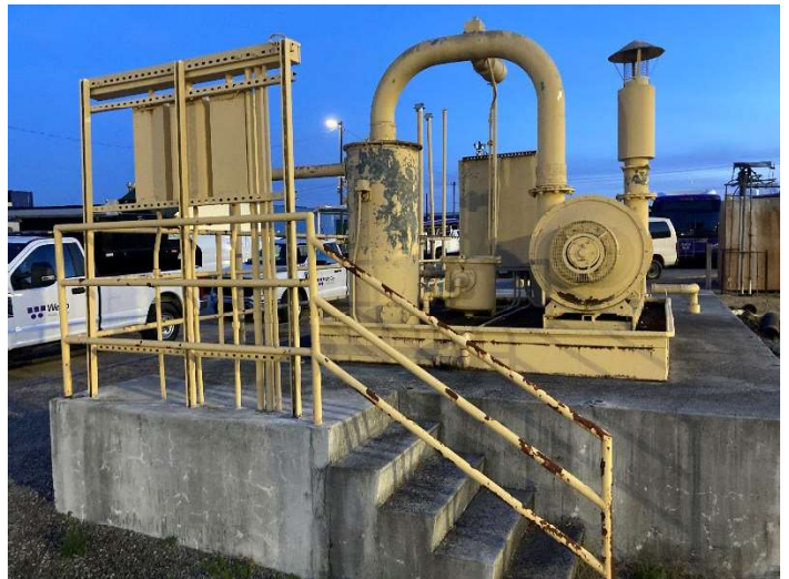
Photo 6: Concrete Pad and Equipment to Be Removed
