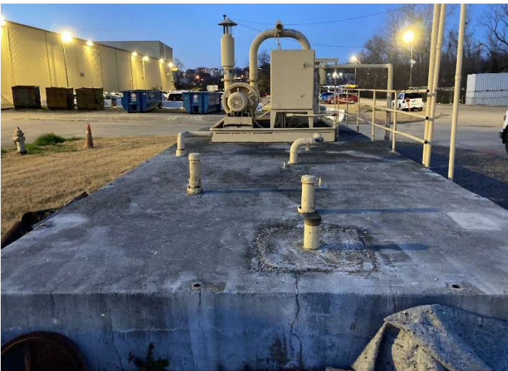
Photo 5: Concrete Pad and Equipment to Be Removed
