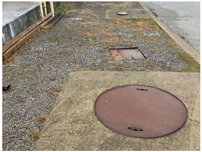
Photo 2: 20,000-Gallon UST (next to concrete slab)
